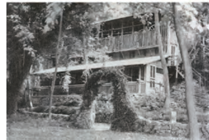
A) Rock Wall Date of Construction: 1921 Materials: Limestone Condition: Good
