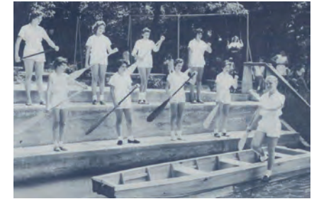
B) Boat Dock Date of Construction: 1923 Materials: Concrete Condition: Fair
