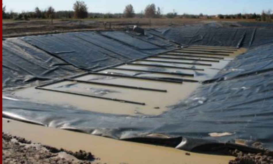
MRPTS vertical flow bioreactor, under construction, fall 2008
