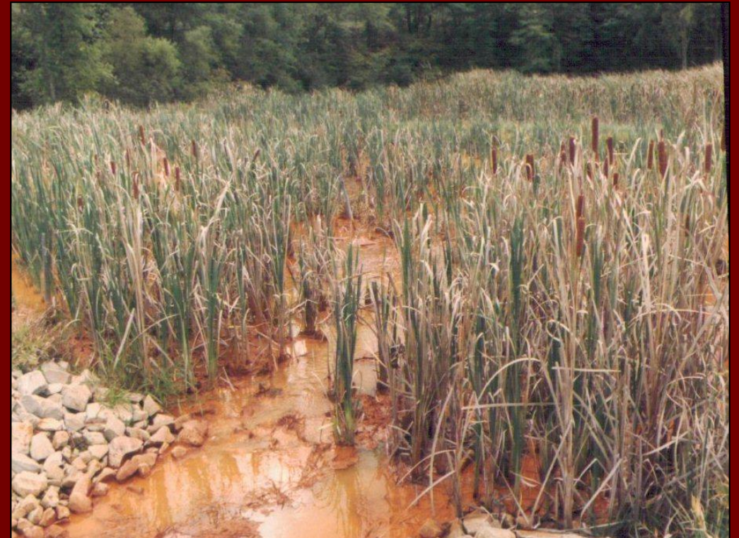
Mine water treatment plants!
