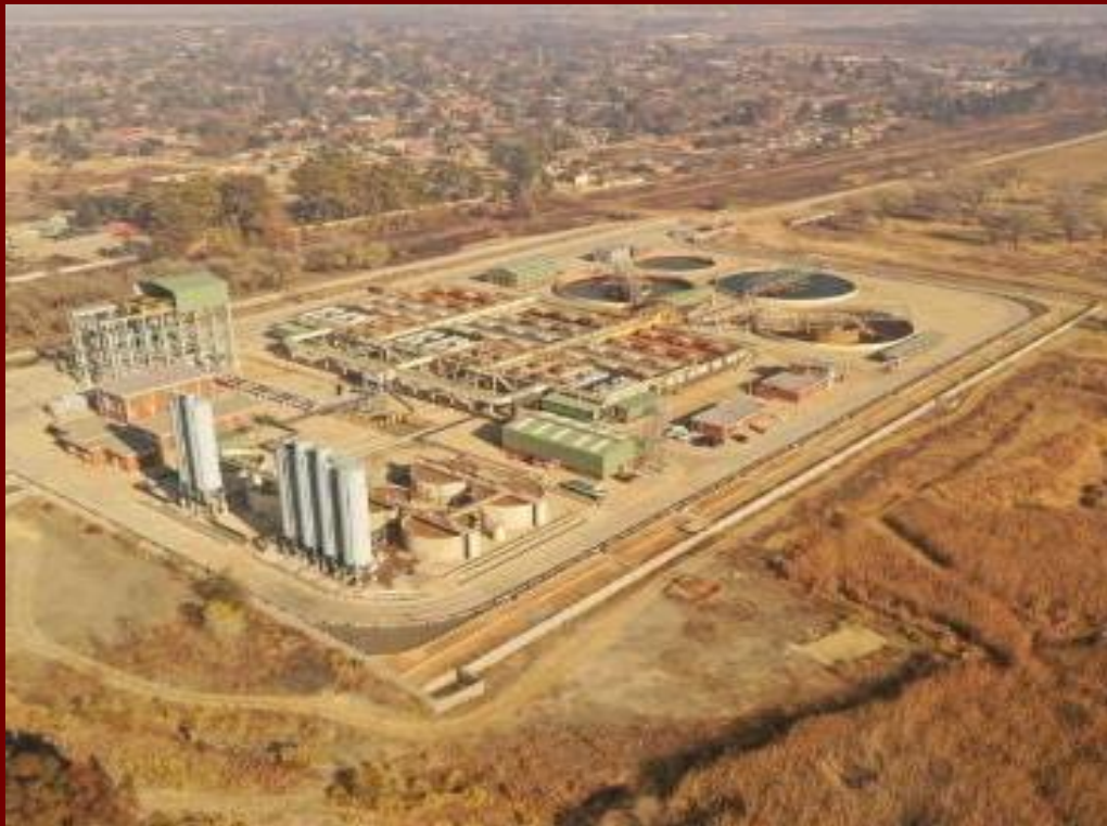
Mine water treatment plant
